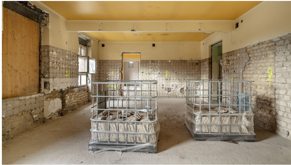
Tiles dismantled and conditioned for transport © Luc Boegly
