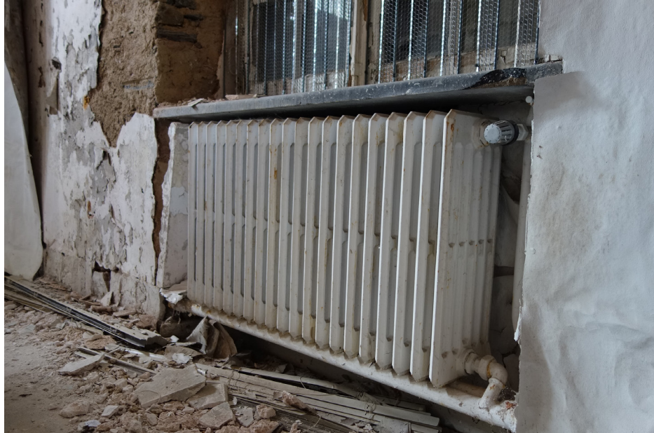
Survey of potentially reusable materials: cast-iron radiator - Wiltz © Rotor
